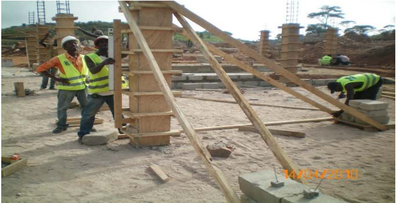
Erection of superstructure columns on Block B
