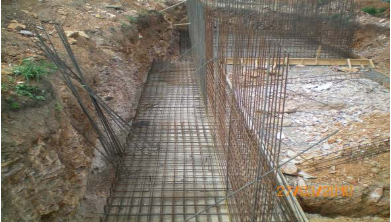
Reinforcement in the retaining wall in basement
