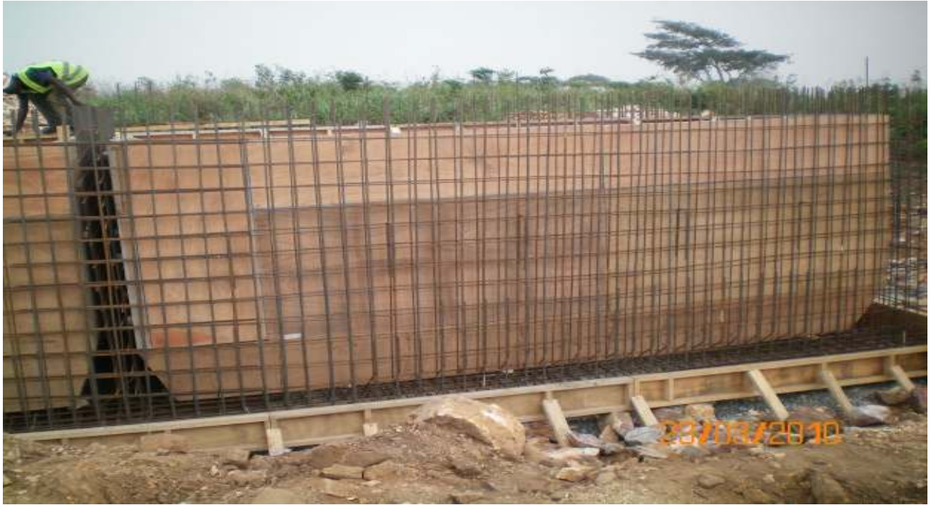
Water tank formwork and reinforcement ready
