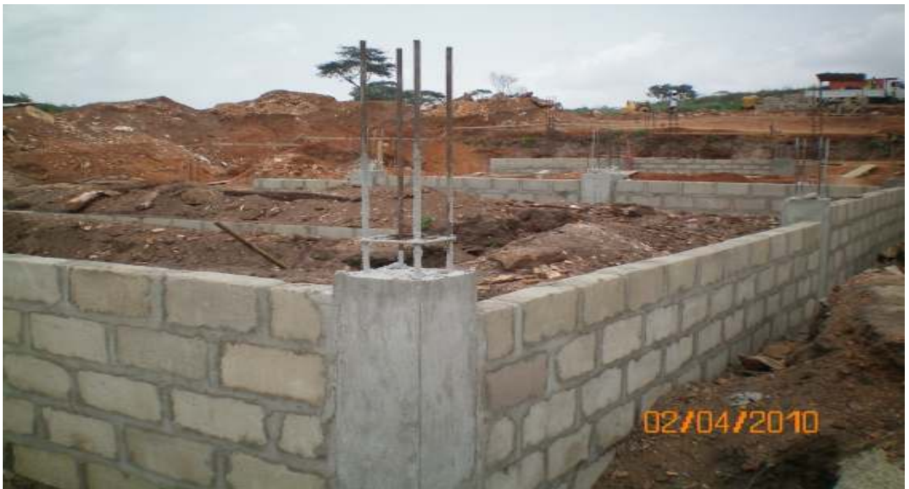
Lecture Hall A substructure works
