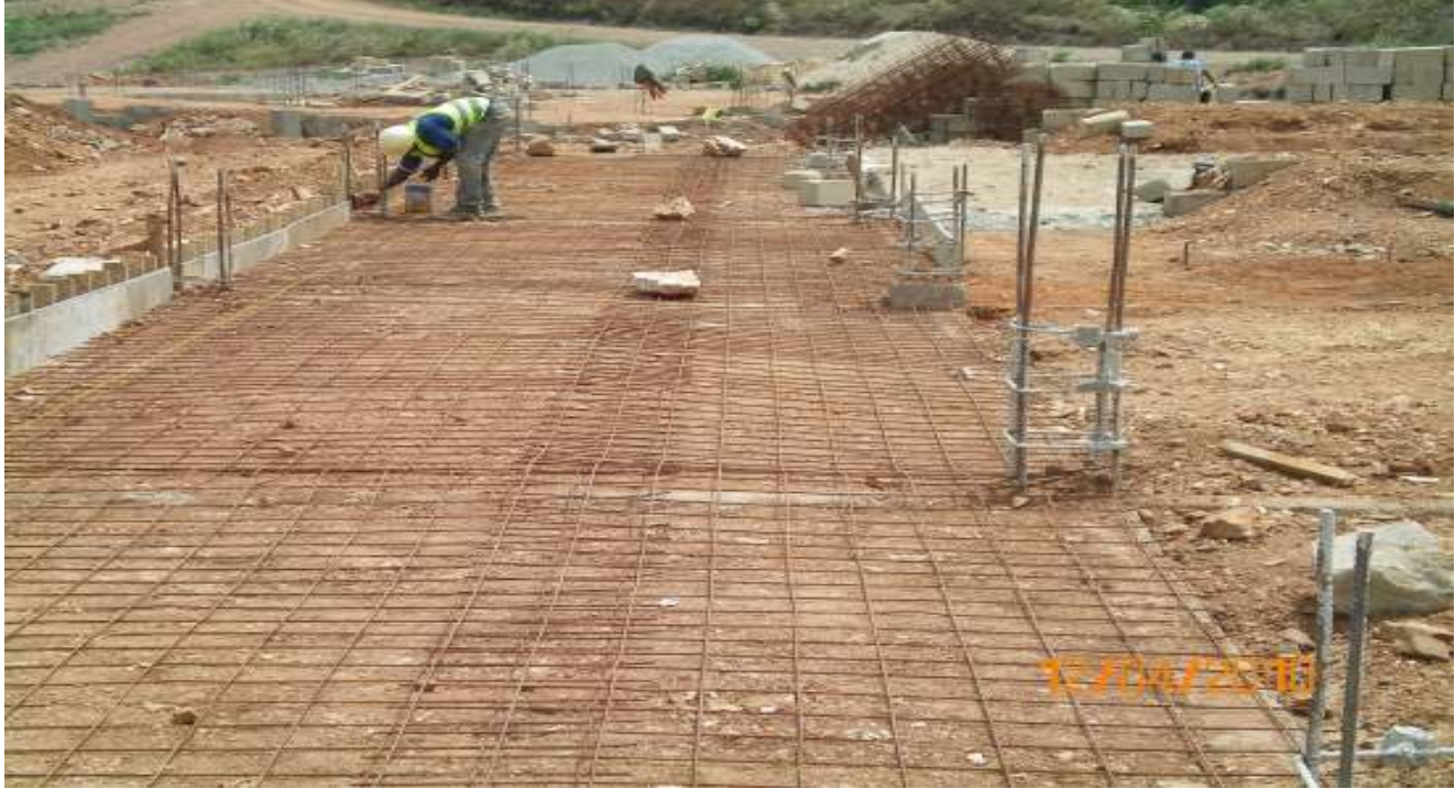
Mesh arrangement in Block C
