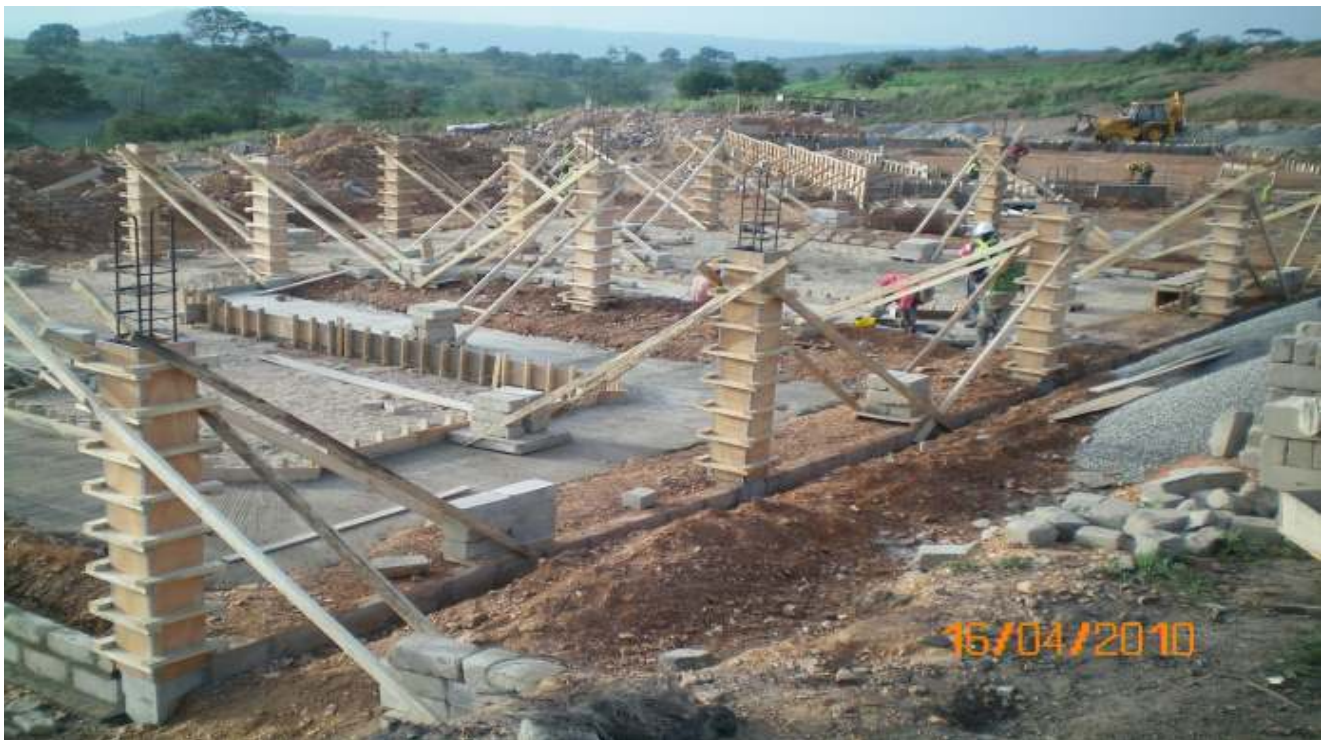
Superstructure columns on Block B
