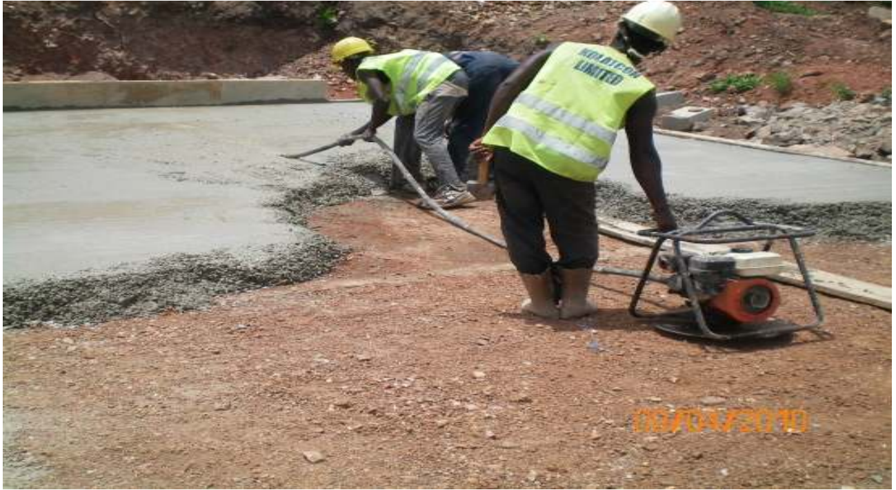
Casting of Block B concrete bed
