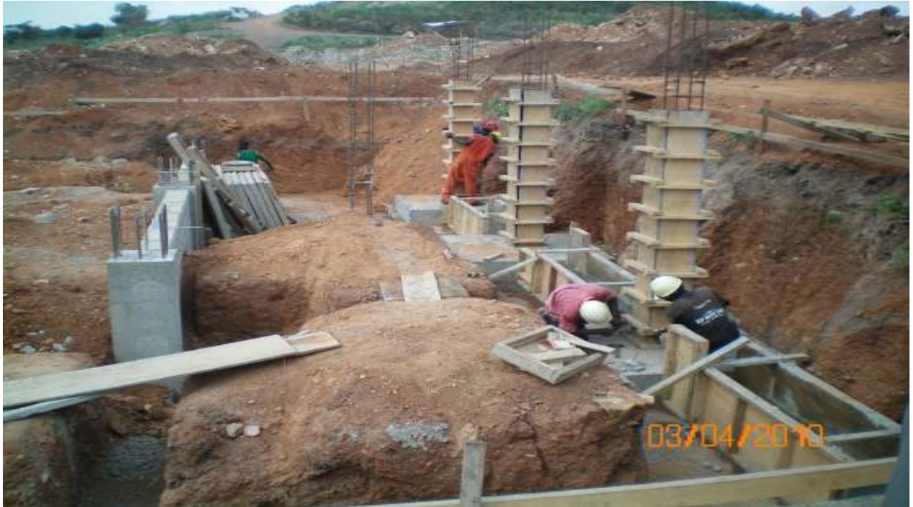
Lecture Hall A substructure works
