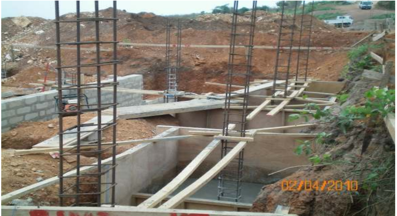
Lecture Hall A substructure works
