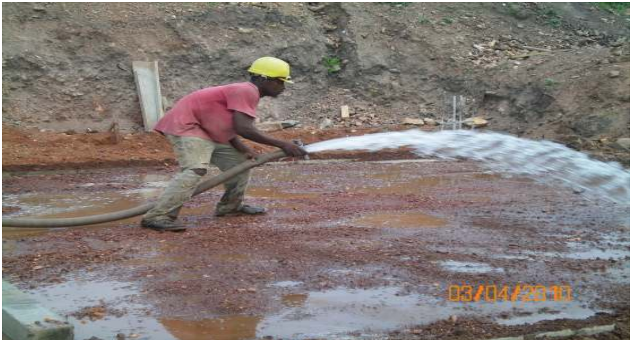
Watering of Block B hardcore fill
