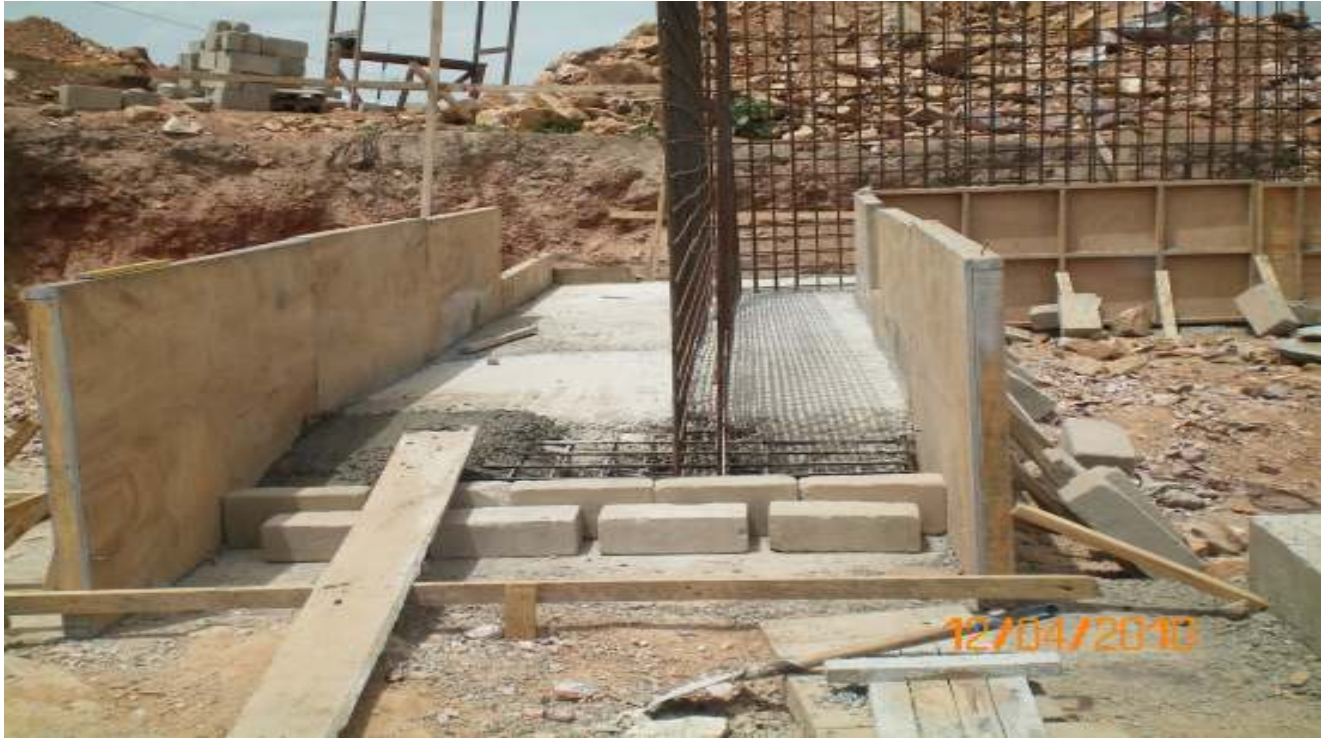
Retaining wall in Administration Block
