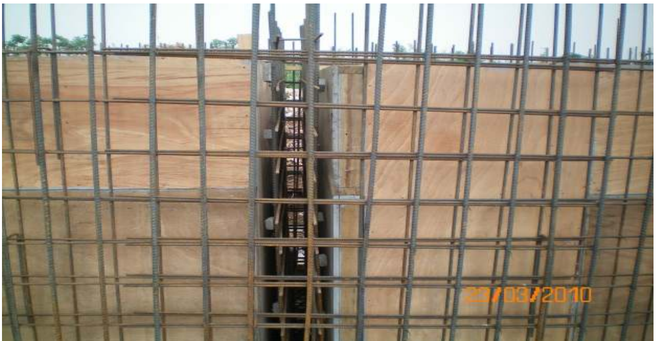
Water tank formwork and reinforcement ready
